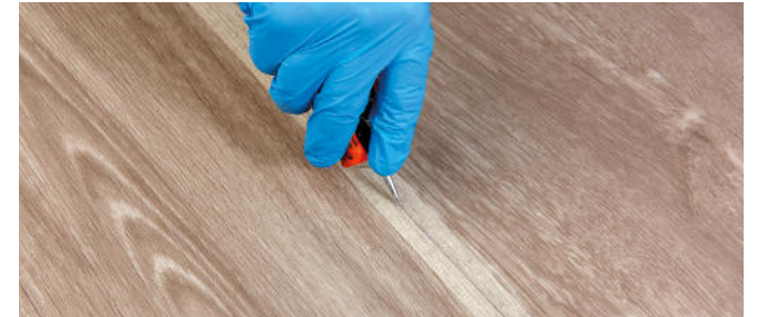
Figure 7 Cold welding
