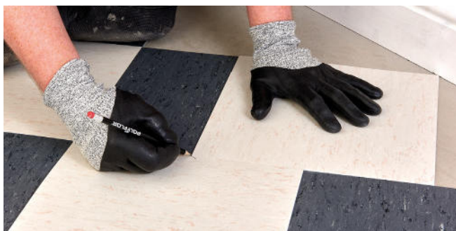
Figure 7 Marking the perimeter tiles (diagonal cut)
