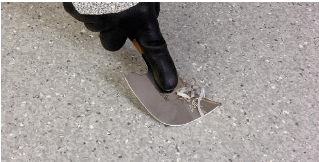
Figure 5a Final trim after the weld has cooled (Spatula Trimming Knife)
