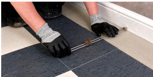
Figure 6 Measuring a tile using a scriber
