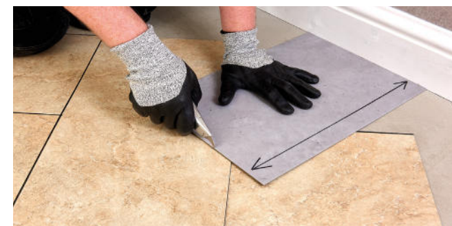
Figure 9 Cutting the perimeter tiles (diagonal cut)
