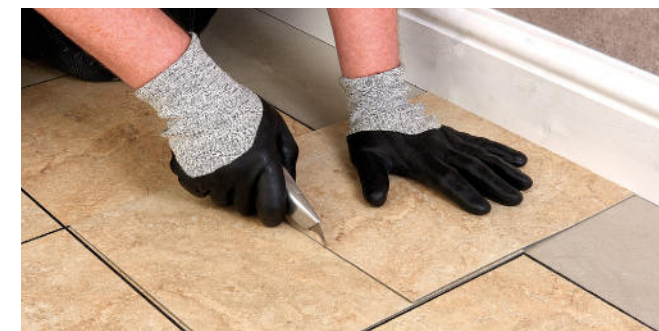
Figure 6 Measuring using an overlapping tile
