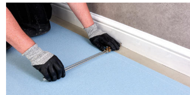
Figure 2 Scribing the wall profile
