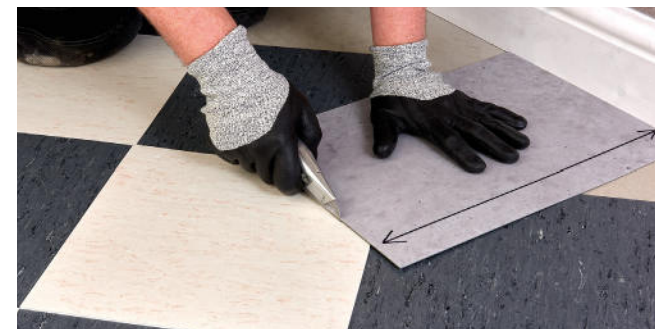
Figure 8 Cutting the perimeter tiles (diagonal cut)
