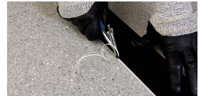
Figure 1 Grooving the seam
