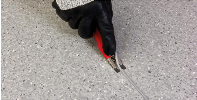
Figure 4b Trimming off the weld top layer (Mozart Trimming Tool)
