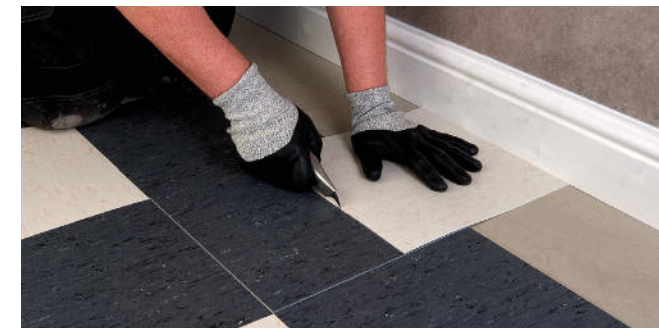
Figure 5 Measuring using an overlapping tile
