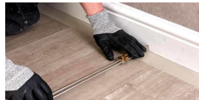
Figure 2 Scribing the wall profile
