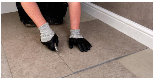
Figure 8 Measuring using an overlapping tile
