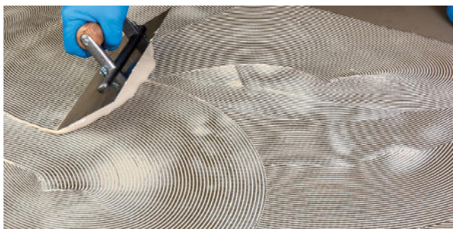
Figure 6 Spread the adhesive
