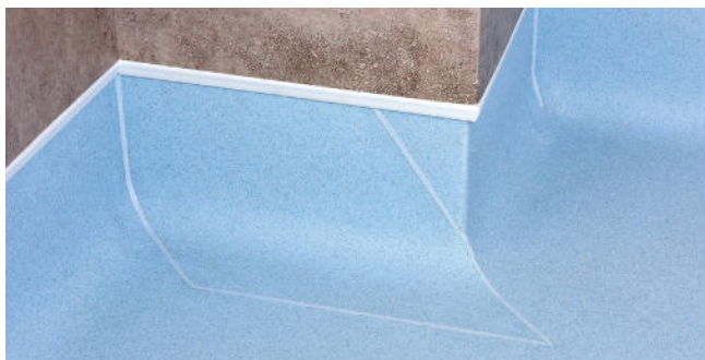
Figure 11 External corners 'wrap around method'
