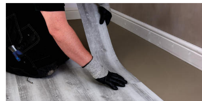
Figure 1 Setting planks out
