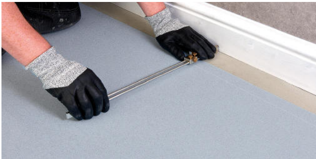
Figure 11 Scribing the wall profile
