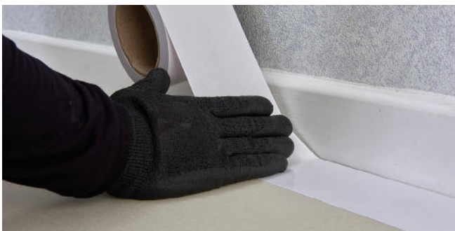
Figure 12 Use double sided Polyflor recommended tape
