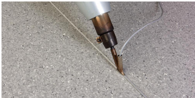
Figure 2 Applying the weld
