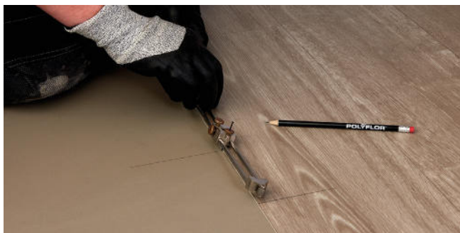
Figure 4 Scribing the wall profile
